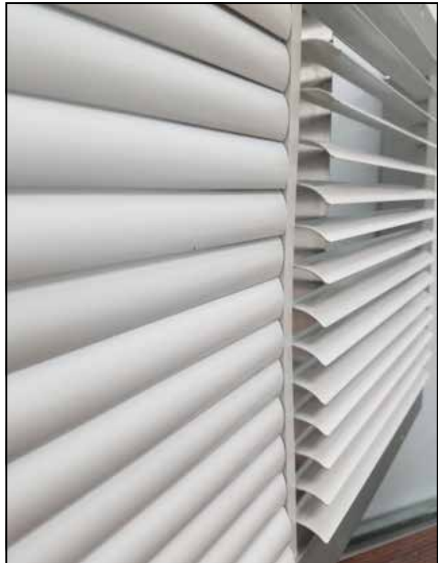
FIGURE 6 Downward Curved Diverter Blades
