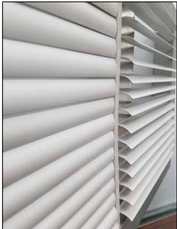
FIGURE 6 Downward Curved Diverter Blades
