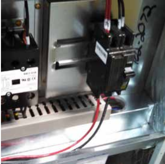
FIGURE 13 Wire Routing
