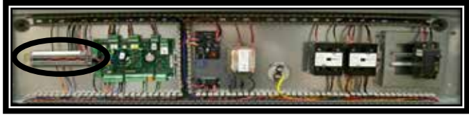
FIGURE 30 Communication Wiring: Termination at the First Wall-Mount Unit
