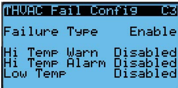
FIGURE 48 Changing HVAC Fail Outputs
