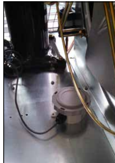
FIGURE 3 Outdoor Sensor Installation
