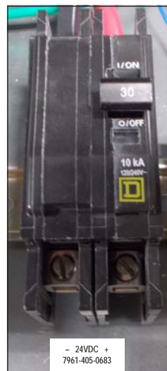
FIGURE 2 VIC1500 Connections Points: Power Supply
