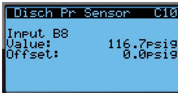
FIGURE 39 Adjusting Discharge/Liquid Transducer Pressure Values
