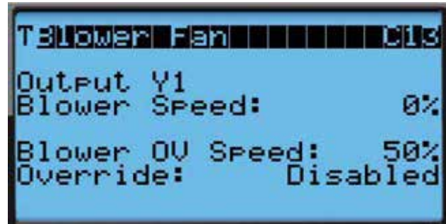
FIGURE 32 Putting Blower Output into Override Mode
