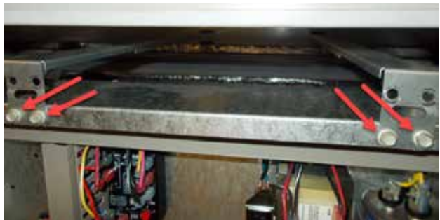
FIGURE 6 Remove Four Screws
