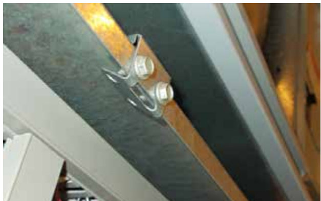
FIGURE 8 Re-Install Screws and Bend Tabs Up
