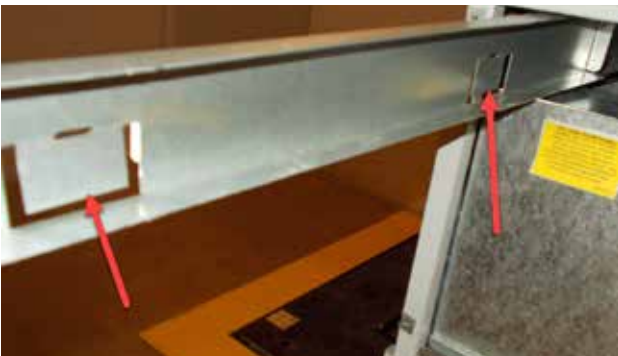
FIGURE 5 Bend Filter Tabs Down
