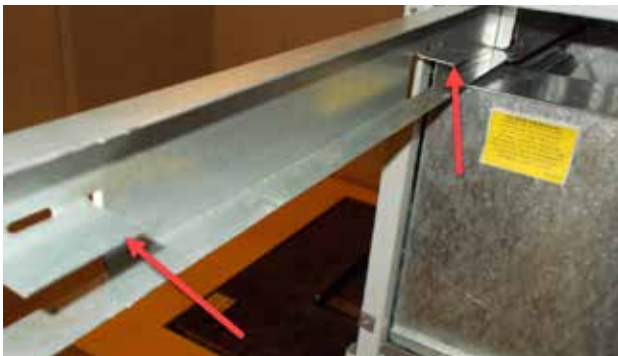
FIGURE 4 Filter Tabs in Up Position
