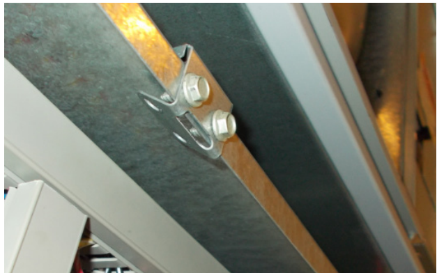
FIGURE 8 Re-Install Screws and Bend Tabs Up
