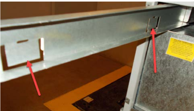
FIGURE 5 Bend Filter Tabs Down
