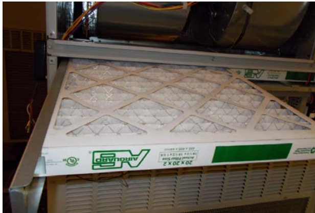
FIGURE 10 Install Left 2" Filter
