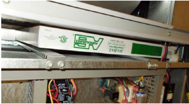
FIGURE 10 Install Left 2" Filter
