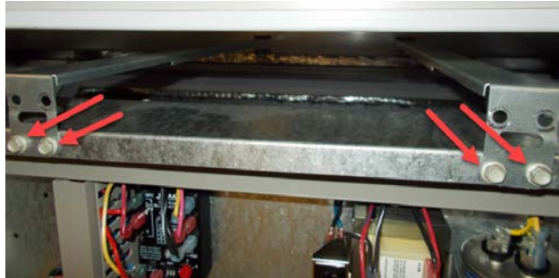
FIGURE 6 Remove Four Screws
