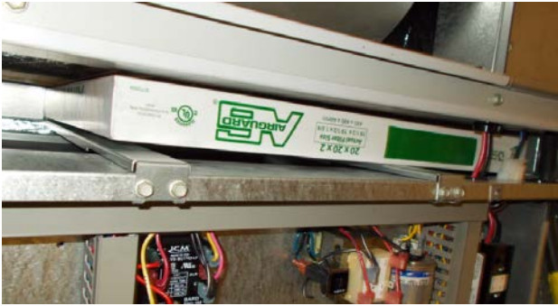
FIGURE 10 Install Left 2" Filter
