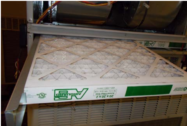
FIGURE 10 Install Left 2" Filter
