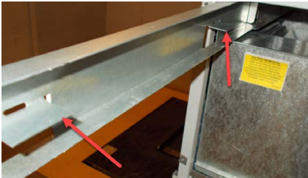
FIGURE 4 Filter Tabs in Up Position
