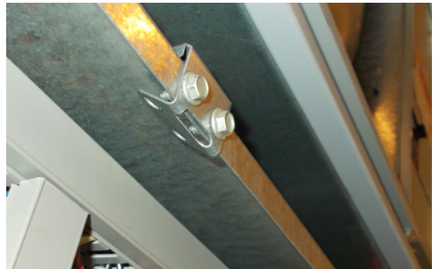
FIGURE 8 Re-Install Screws and Bend Tabs Up
