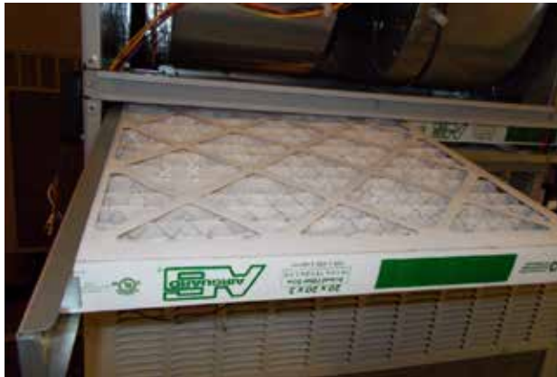
FIGURE 10 Install Left 2" Filter
