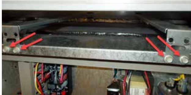
FIGURE 6 Remove Four Screws
