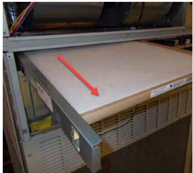
FIGURE 2 Removing Left Filter
