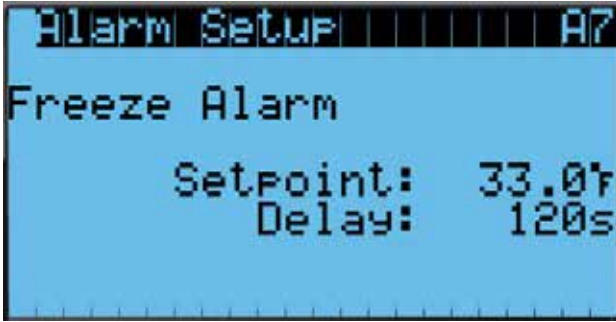
FIGURE 28 Adjusting Freeze Setpoint and Alarm Delay
