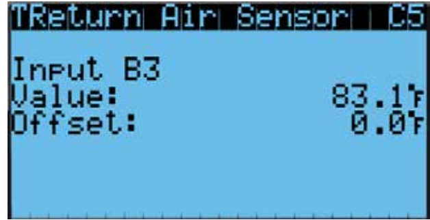
FIGURE 18 Adjusting Return Air Sensor
