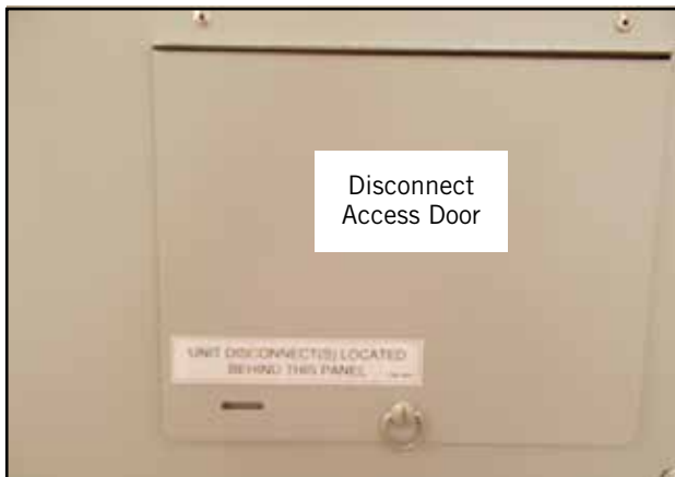
FIGURE 1 Disconnect Power
