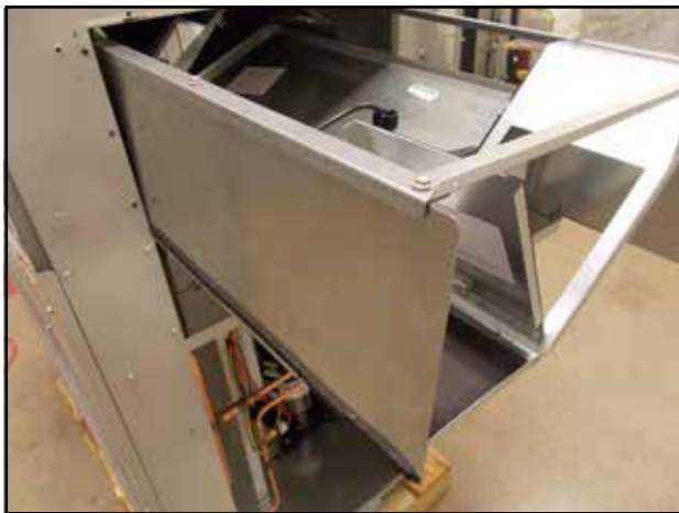
FIGURE 10 Install Vent
