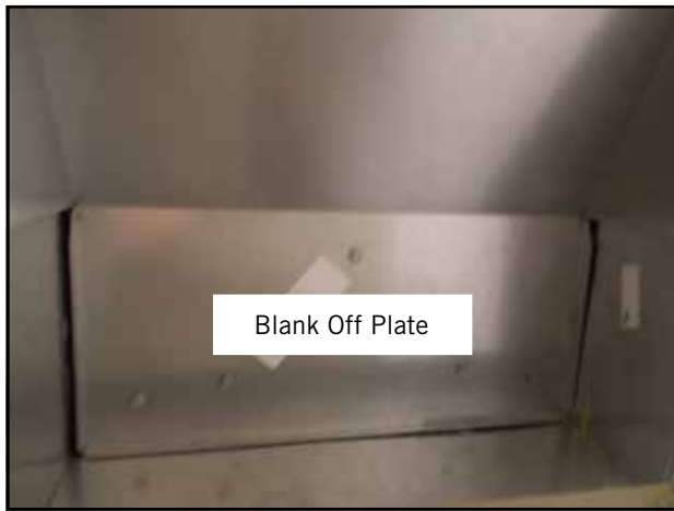
FIGURE 4 Remove Blank Off Plates (Both Sides)
