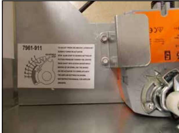
FIGURE 14 Set Blade Stop to Adjust Fresh Air Amount
