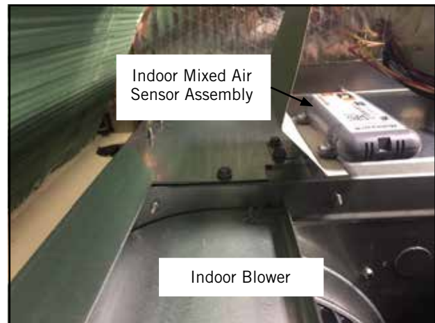
FIGURE 11 Install Indoor Mixed Air Sensor Assembly
