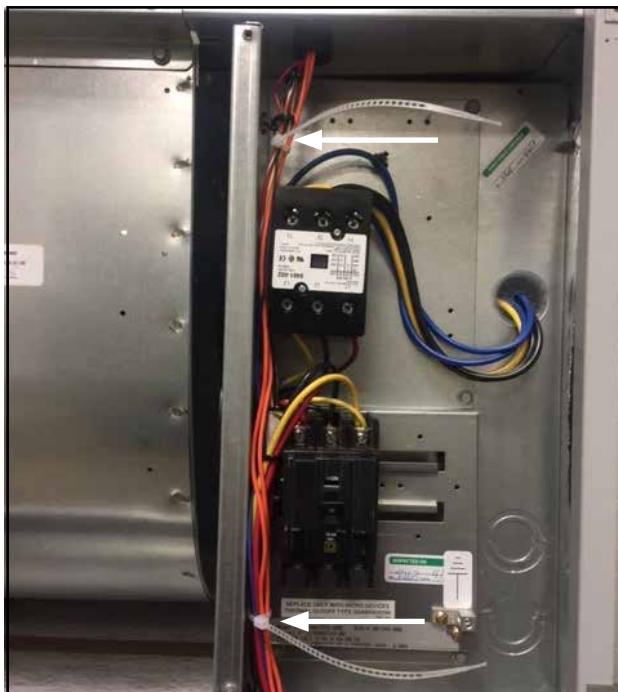
FIGURE 13 Secure Sensor Wires with Ladder Ties
