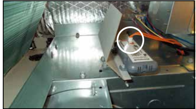
FIGURE 14 Connect Mixed Air Sensor Plug
