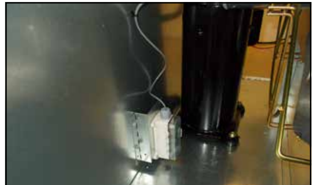
FIGURE 15 Enthalpy Sensor Assembly Installation
