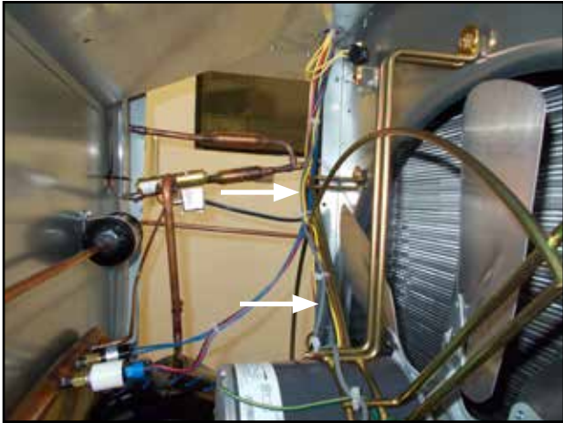
FIGURE 17 Route Wires and Secure with Ties
