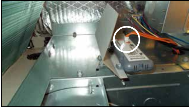
FIGURE 16 Connect Mixed Air Sensor Plug
