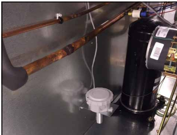
FIGURE 18 Temperature Only Sensor Assembly Installation
