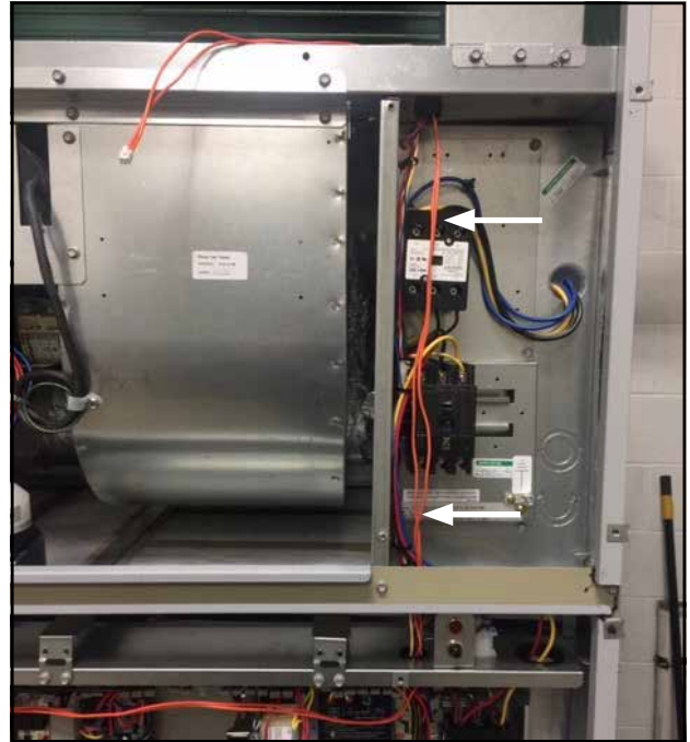
FIGURE 14 Route Orange Mixed Air Sensor Wires
