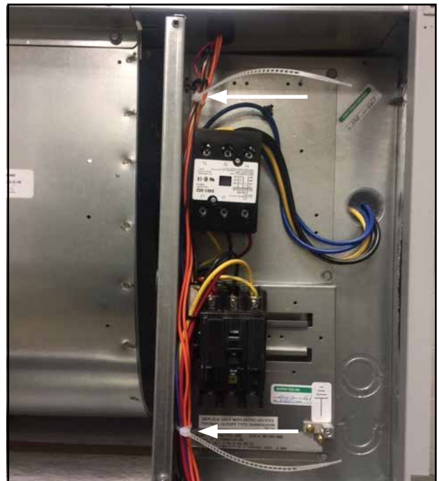
FIGURE 15 Secure Sensor Wires with Ladder Ties
