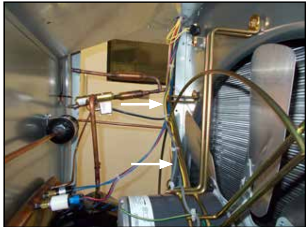
FIGURE 19 Route Wires and Secure with Ties
