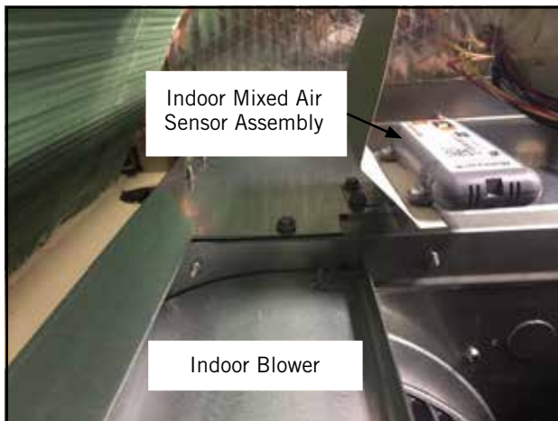
FIGURE 13 Install Indoor Mixed Air Sensor Assembly
