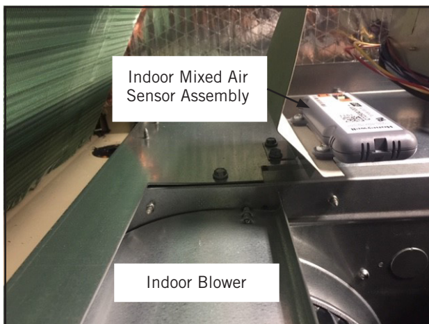
FIGURE 13 Install Indoor Mixed Air Sensor Assembly
