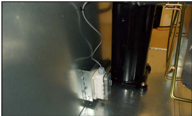
FIGURE 17 Enthalpy Sensor Assembly Installation
