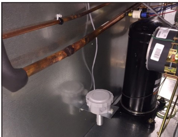
FIGURE 18 Temperature Only Sensor Assembly Installation
