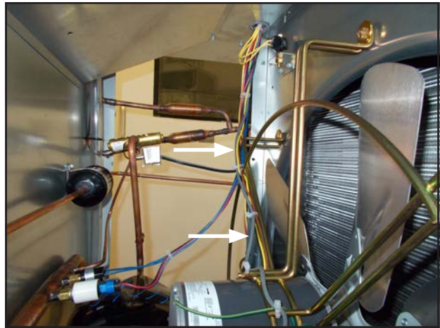
FIGURE 19 Route Wires and Secure with Ties
