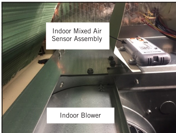
FIGURE 13 Install Indoor Mixed Air Sensor Assembly
