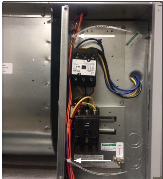
FIGURE 15 Secure Sensor Wires with Ladder Ties
