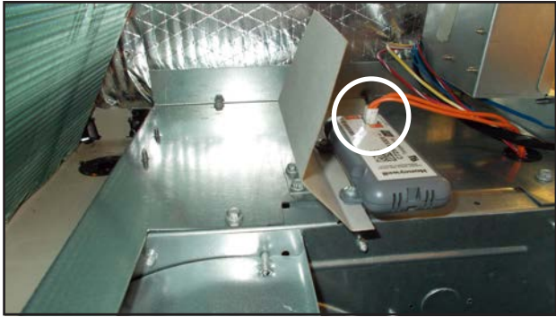
FIGURE 16 Connect Mixed Air Sensor Plug
