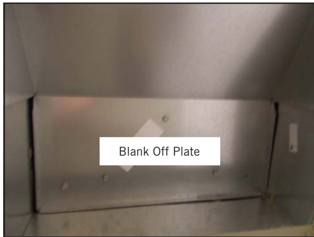
FIGURE 4 Remove Blank Off Plates (Both Sides)
