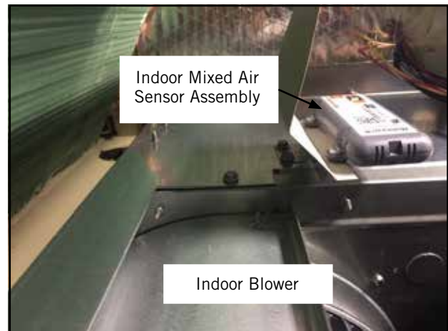
FIGURE 11 Install Indoor Mixed Air Sensor Assembly
