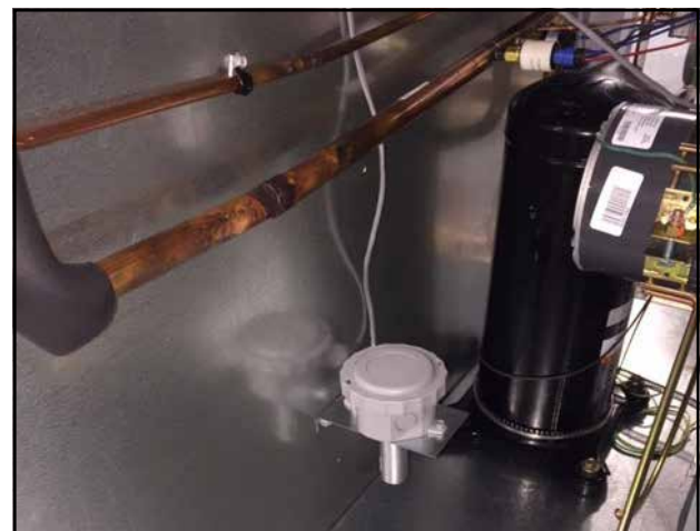
FIGURE 16 Temperature Only Sensor Assembly Installation
