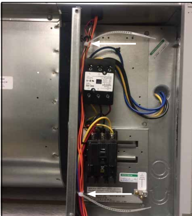
FIGURE 13 Secure Sensor Wires with Ladder Ties
