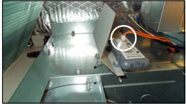
FIGURE 14 Connect Mixed Air Sensor Plug
