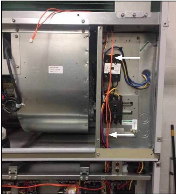
FIGURE 12 Route Orange Mixed Air Sensor Wires
