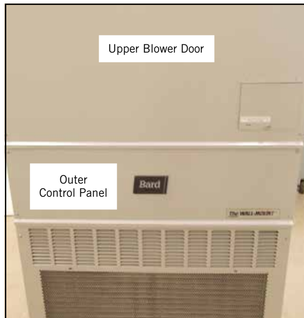
FIGURE 3 Remove Blower Door and Control Panel
