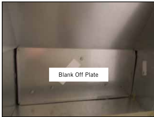
FIGURE 4 Remove Blank Off Plates (Both Sides)
