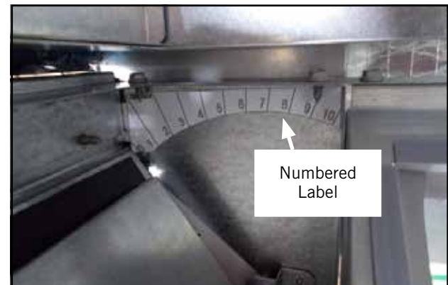
FIGURE 16 Ventilation Air Label
