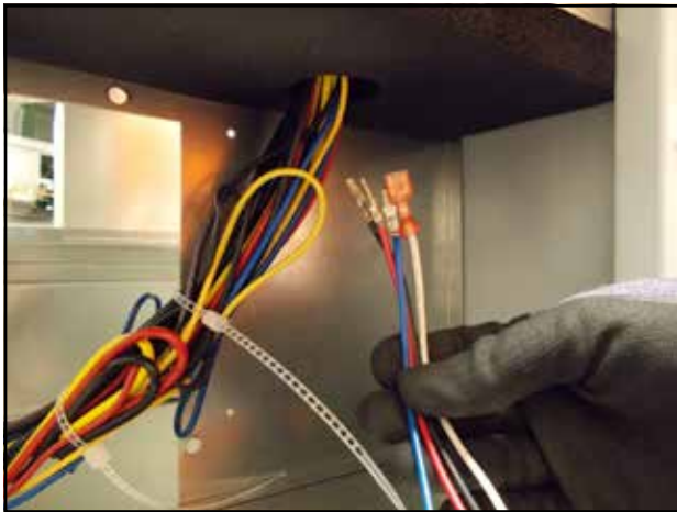
FIGURE 17 Run Wires Up to Control Panel
