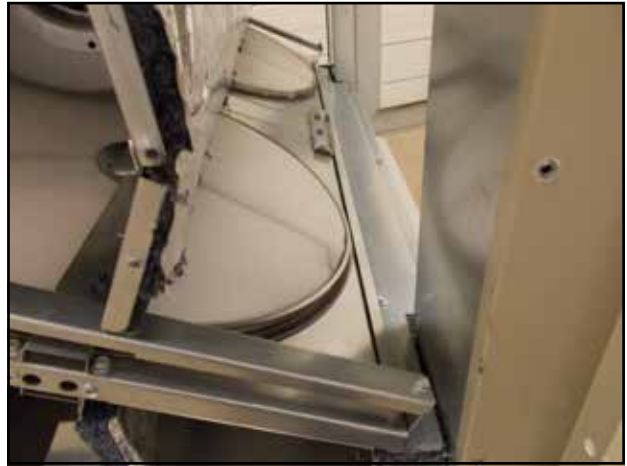
FIGURE 27 Upper Blower Assembly Installed
