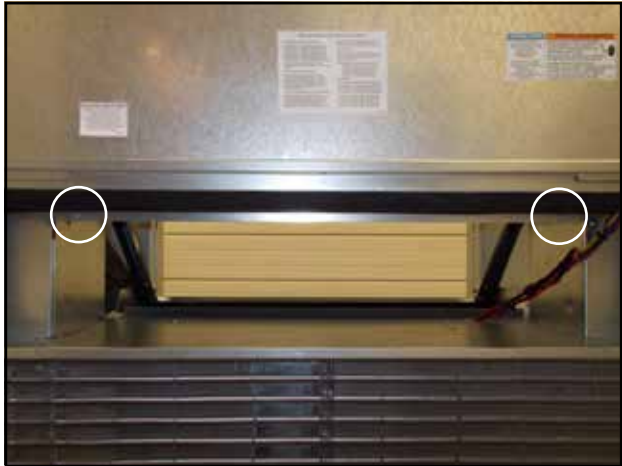
FIGURE 10 Remove Screws from Under Control Panel
