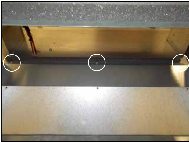
FIGURE 8 Remove Screws from Condenser Partition Insert
