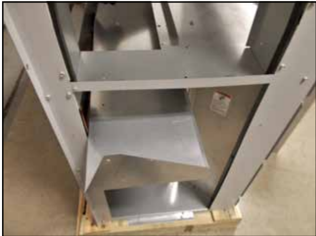
FIGURE 9 Remove Condenser Partition Insert
