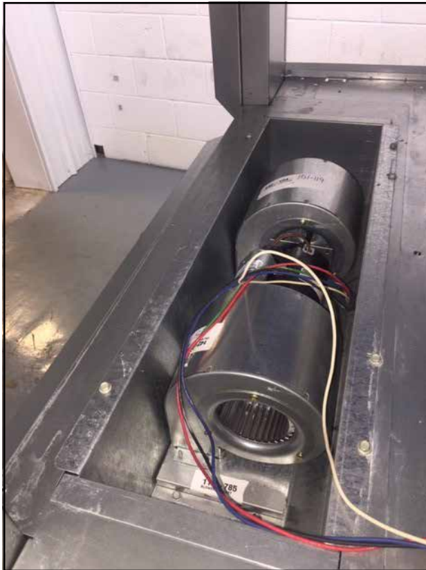
FIGURE 13 Install Exhaust Blower
