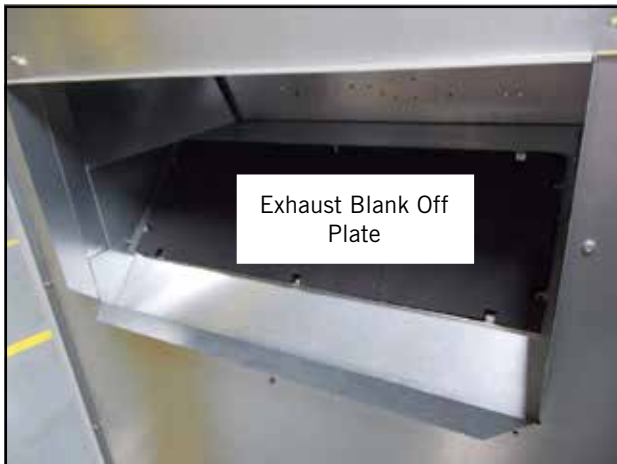
FIGURE 5 Remove Exhaust Blank Off Plate
