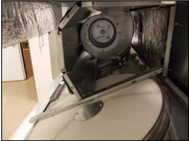
FIGURE 26 Upper Blower Assembly Over Cassettes
