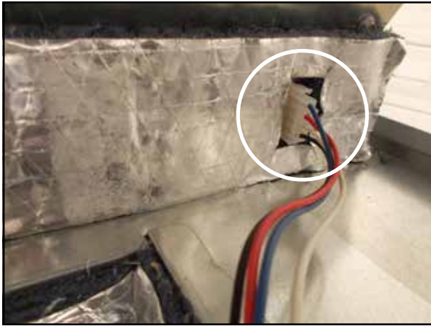
FIGURE 16 Install Exhaust Blower Plug
