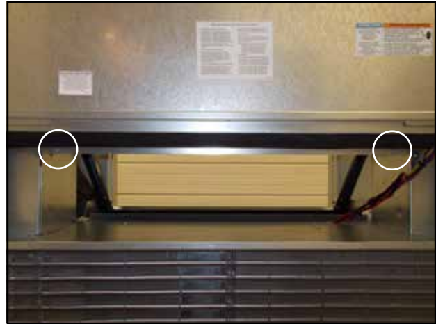
FIGURE 10 Remove Screws from Under Control Panel
