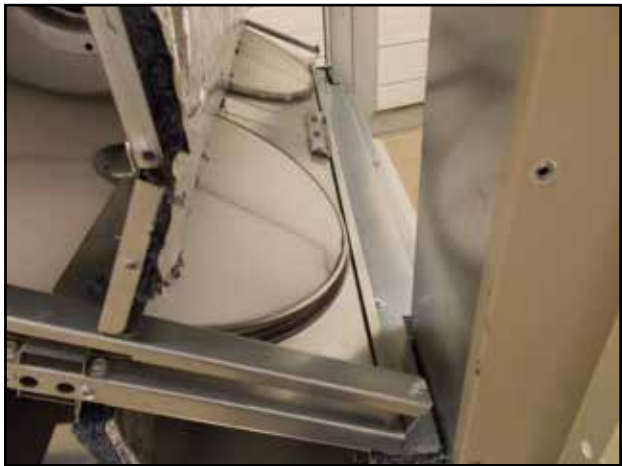
FIGURE 27 Upper Blower Assembly Installed
