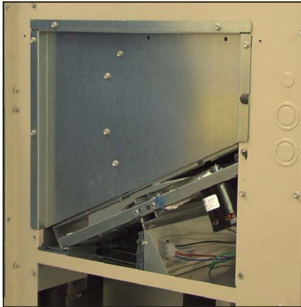
FIGURE 43 Install Upper Side Covers
