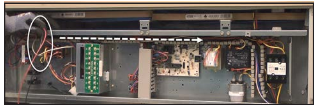
FIGURE 37 Route Red and Black Wires to Compressor Contactor
