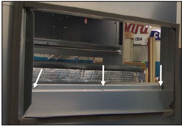
FIGURE 28 Install Rear ERV Mounting Rail
