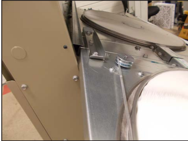
FIGURE 30 Slide Cassette Frame into Mounting Rails
