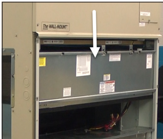
FIGURE 3 Remove Low Voltage Control Panel
