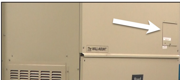
FIGURE 1 Disconnect Power
