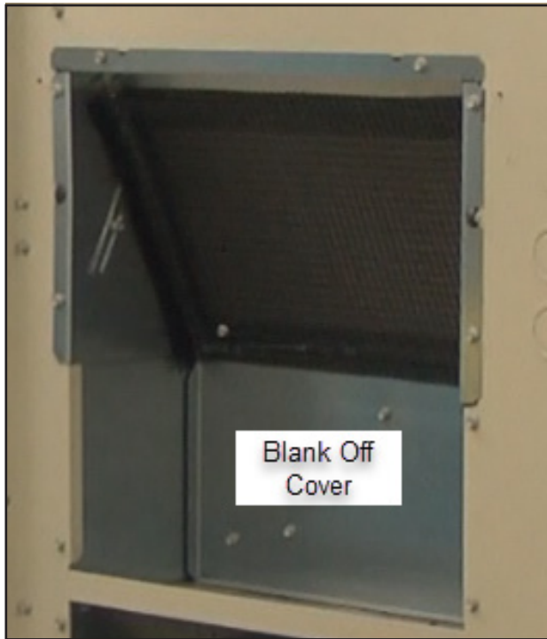
FIGURE 4 Remove Blank Off Covers
