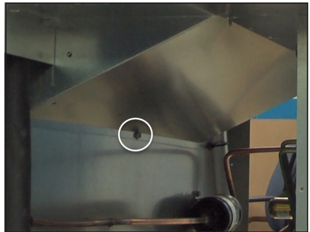
FIGURE 7 Remove Screw from Condenser Partition Insert
