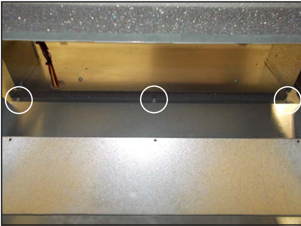
FIGURE 8 Remove Screws from Condenser Partition Insert
