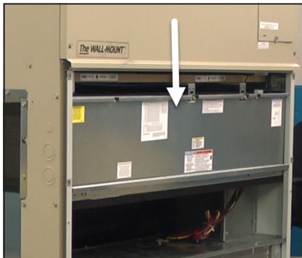
FIGURE 3 Remove Low Voltage Control Panel
