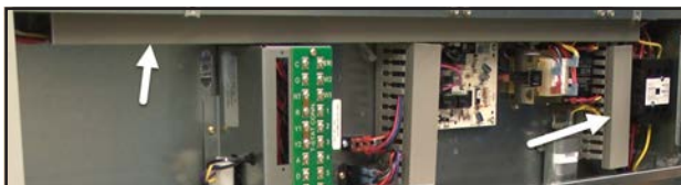
FIGURE 23 Remove Two Wire Channel Covers
