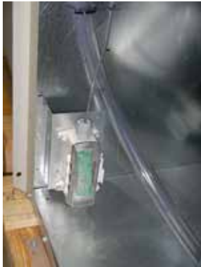
FIGURE 5 Outdoor Air Sensor Installation
