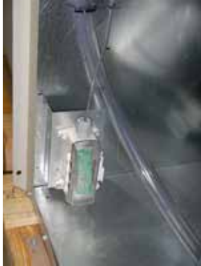
FIGURE 5 Outdoor Air Sensor Installation
