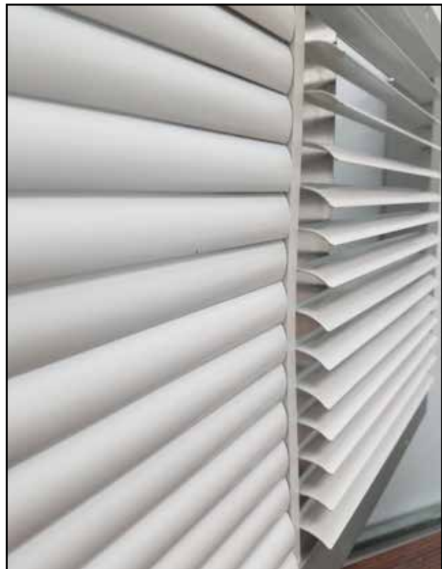
FIGURE 6 Downward Curved Diverter Blades
