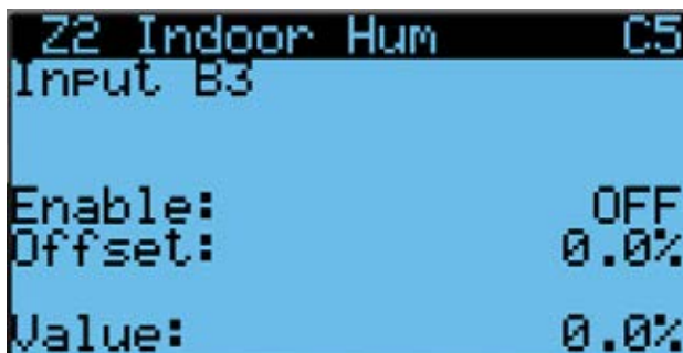
FIGURE 45 Enable/Disable Zone 2 Indoor Humidity Sensor
