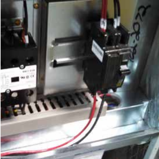
FIGURE 13 Wire Routing
