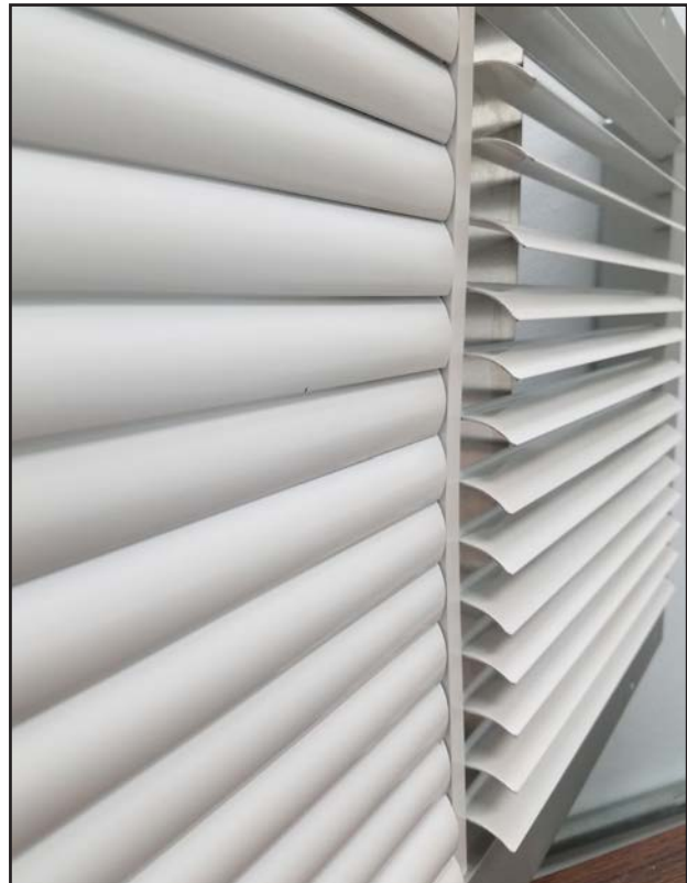
FIGURE 6 Downward Curved Diverter Blades
