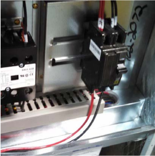
FIGURE 16 Side Communication and Power Wire Entrances (Recommended)
