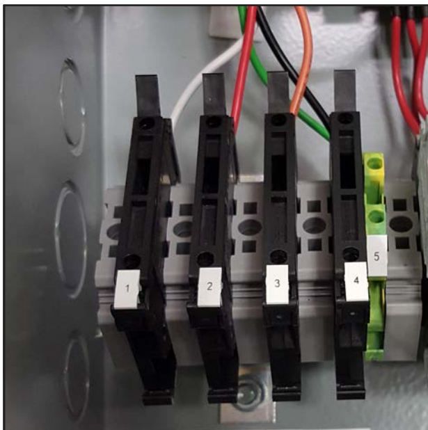
FIGURE 21 LC6000 Fused Power Supply Terminals
