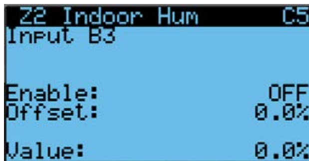
FIGURE 37 Enable/Disable Zone 2 Indoor Humidity Sensor
