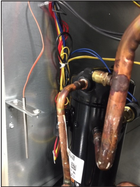
FIGURE 6 Outdoor Air Sensor Installation
