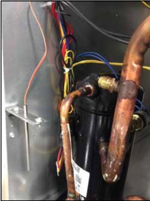
FIGURE 5 Outdoor Air Sensor Installation
