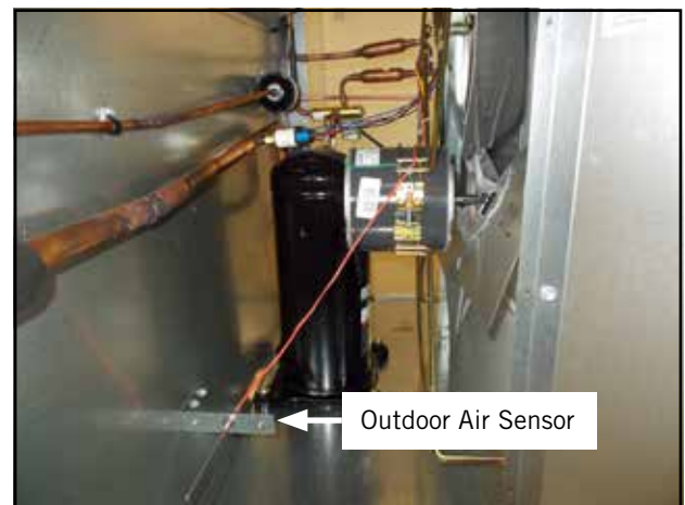
FIGURE 7 Install Outdoor Air Sensor
