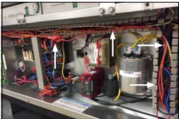
FIGURE 11 Route Wires into Wire Channel and Connect to Wire Harness
