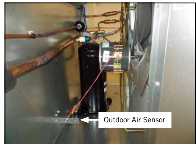
FIGURE 7 Install Outdoor Air Sensor
