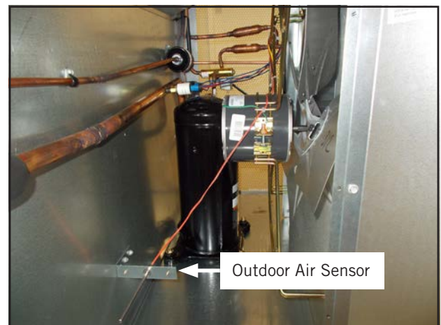
FIGURE 7 Install Outdoor Air Sensor
