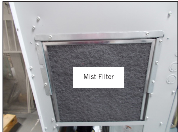
FIGURE 19 Install Mist Filters
