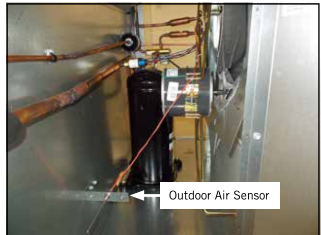
FIGURE 7 Install Outdoor Air Sensor
