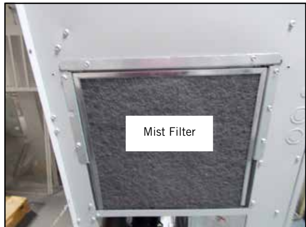
FIGURE 19 Install Mist Filters
