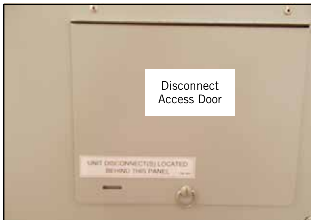
FIGURE 1 Disconnect Power
