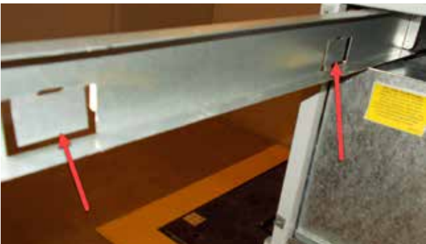
FIGURE 5 Bend Filter Tabs Down
