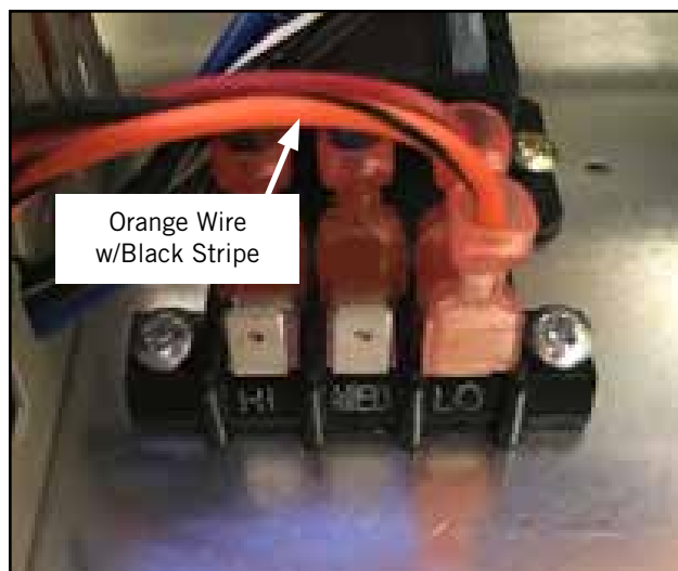
FIGURE 28 Speed Taps
