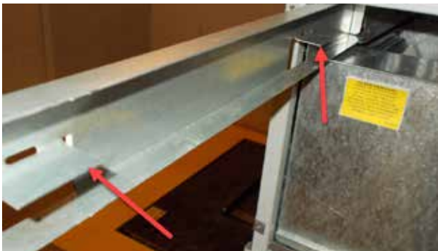
FIGURE 4 Filter Tabs in Up Position
