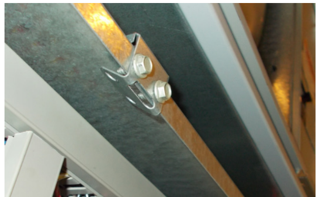
FIGURE 8 Re-Install Screws and Bend Tabs Up
