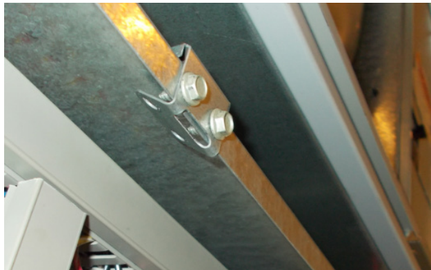
FIGURE 8 Re-Install Screws and Bend Tabs Up
