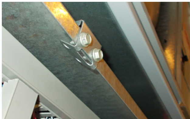
FIGURE 8 Re-Install Screws and Bend Tabs Up
