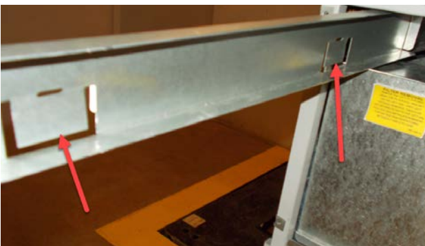
FIGURE 5 Bend Filter Tabs Down
