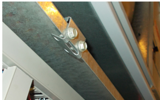
FIGURE 8 Re-Install Screws and Bend Tabs Up
