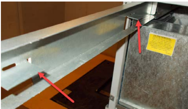
FIGURE 4 Filter Tabs in Up Position
