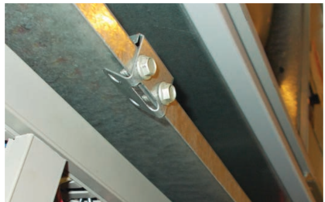
FIGURE 8 Re-Install Screws and Bend Tabs Up
