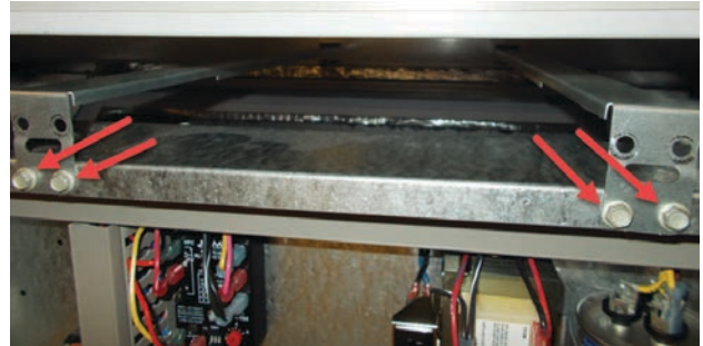
FIGURE 6 Remove Four Screws
