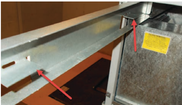
FIGURE 4 Filter Tabs in Up Position
