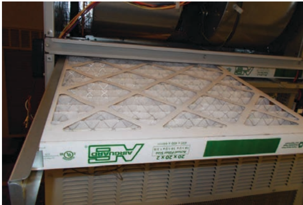
FIGURE 10 Install Left 2" Filter
