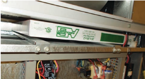
FIGURE 10 Install Left 2" Filter
