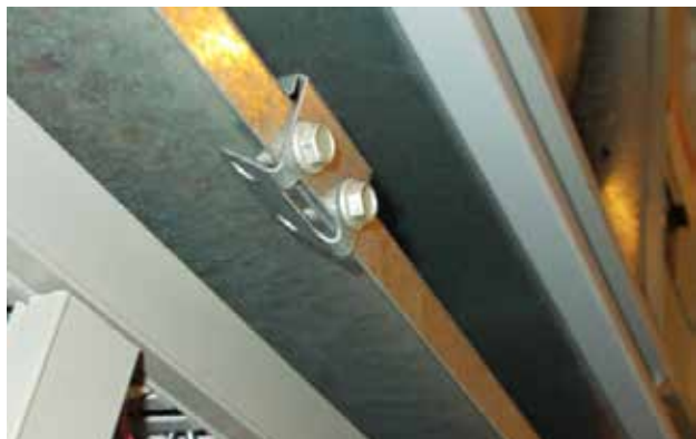
FIGURE 8 Re-Install Screws and Bend Tabs Up
