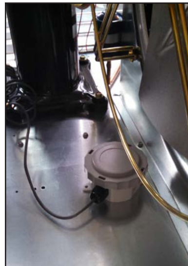
FIGURE 3 Outdoor Sensor Installation
