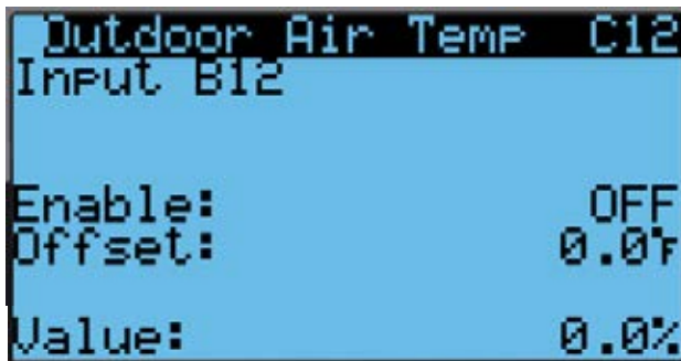
FIGURE 42 Enable/Disable Outdoor Air Temperature
