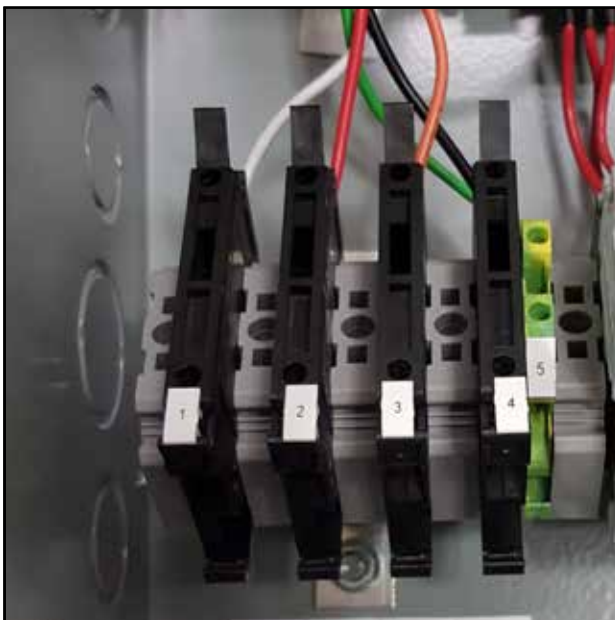
FIGURE 13 LC6000 Fused Power Supply Terminal
