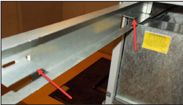
FIGURE 4 Filter Tabs in Up Position
